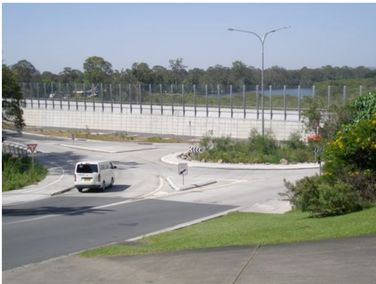
Photo 3.2 View from Rajah Road across the northern approach to the Brunswick River showing the benefit of the clear noise barriers in maintaining the local visual amenity.
