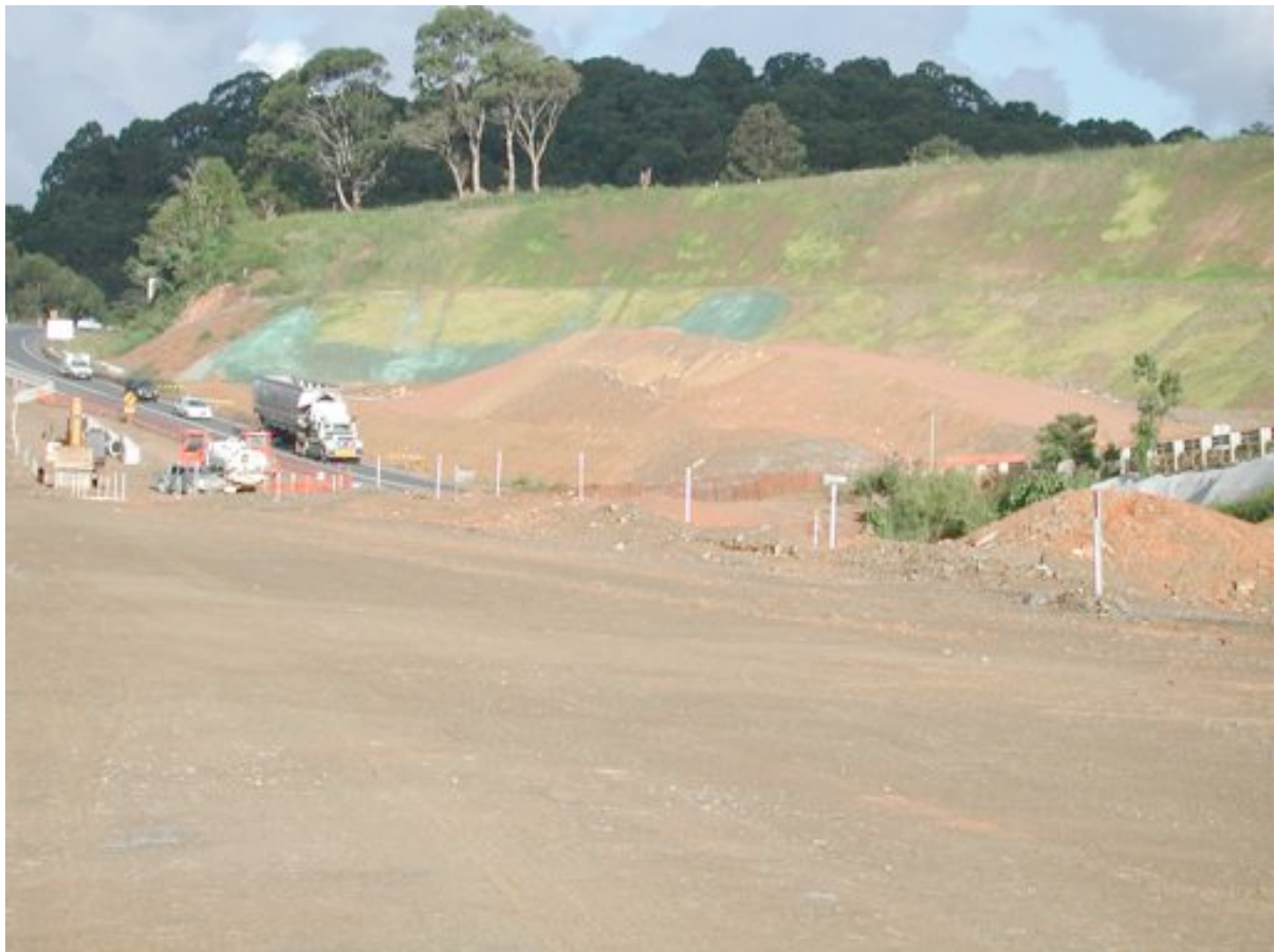
Photograph 3.33 Progressive stabilisation of batters at the Yelgun Rest Area.
