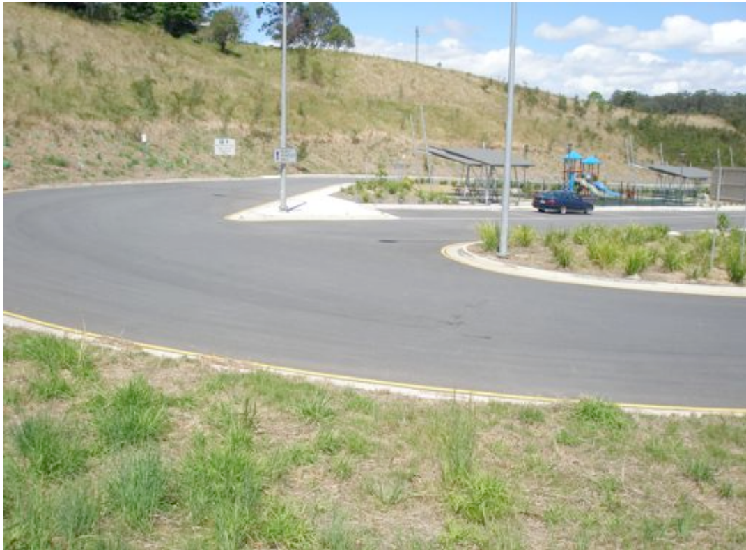
Photograph 3.34 The stabilised batters at the Yelgun Rest Area. The vegetation appears brown as a consequence of recent mowing.
