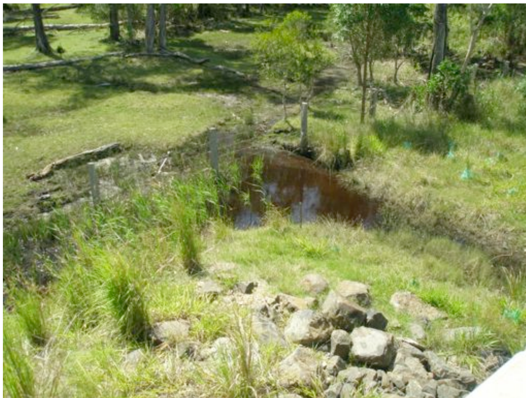
Photograph 3.35 Stabilised wetland at southern end of Upgrade.
