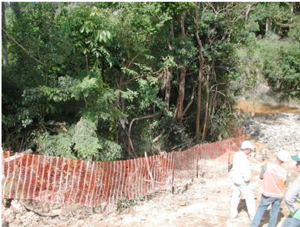
Photograph 3.20 'Paraweb' fencing delineating clearing zone.
