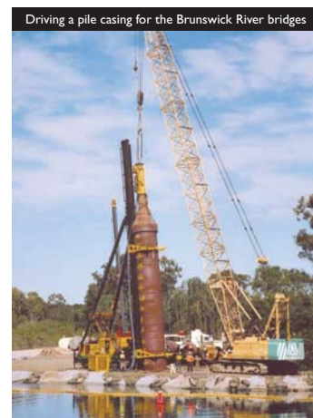
Driving a pile casing for the Brunswick River bridges
