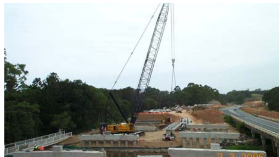
Above: Marshalls Creek bridge deck
