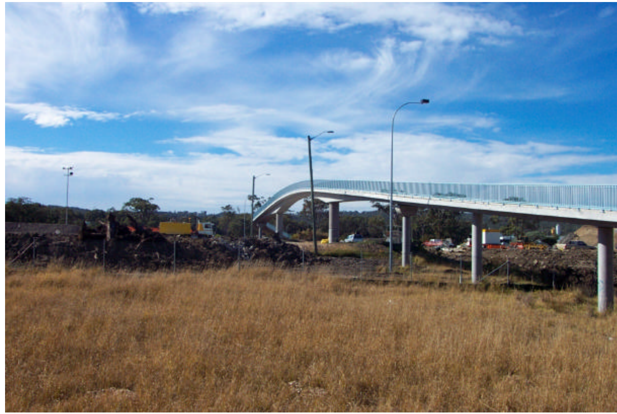
Pedestrian overbridge Charlestown Bypass
